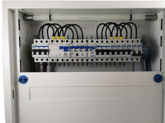
Correct installation position
